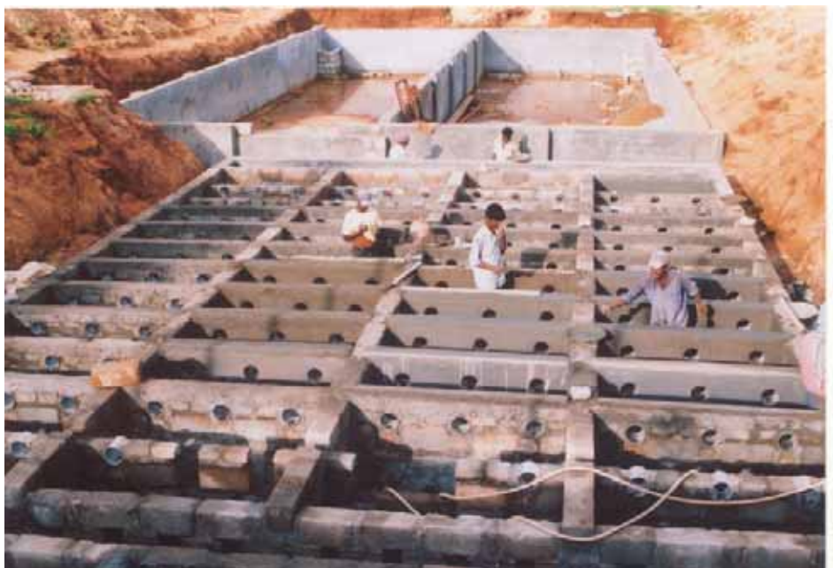
Construction of an anaerobic baffled reactor
