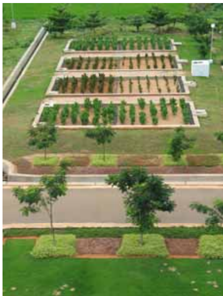
Left: Planted Gravel Filter – Below: construction & design draft of the DEWATS system for the Aravind Eye Hospital - Right: Kim Bang District Hospital, Vietnam
