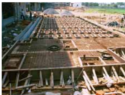
DEWATS polishing pond at a Hotel in Cochin, India (above) – DEWATS under construction (below)
