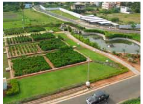
Planted gravel filter and polishing pond in the garden of the Aravind Eye Hospital, India
