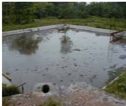
Open disposal can overflow in heavy rains causing runaway spread of diseases
