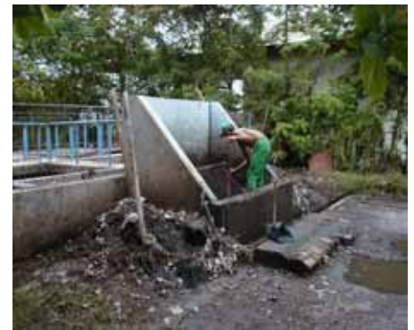
Neglected maintenance contradicts original intentions and design of sanitary facilities
