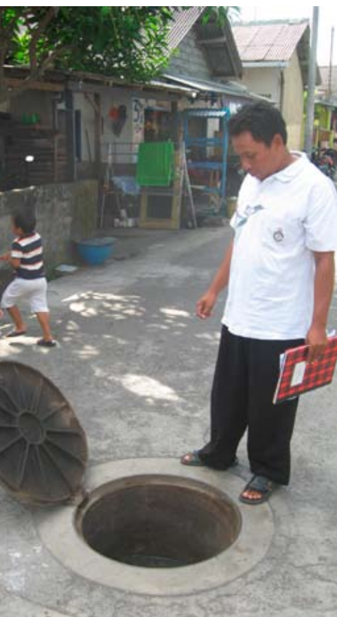
Construction of a DEWATS for a CBS/ SANIMAS project in a small settlement in Mojokerto, East Java
